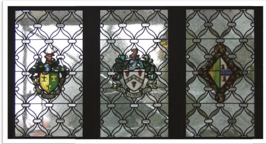
Figure 3-Stone set stained glass windows after restoration
