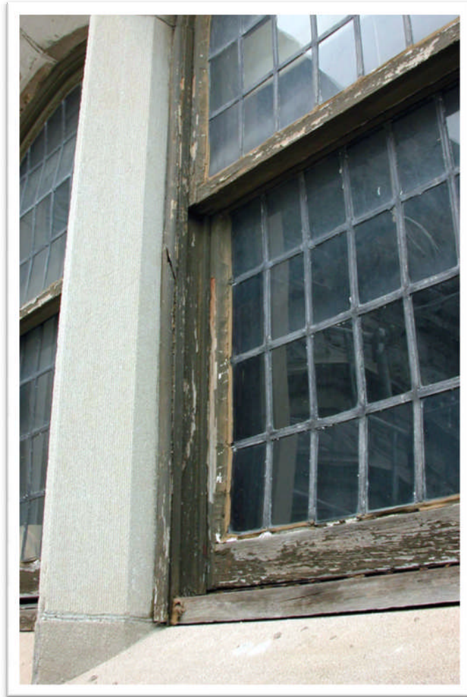
Figure 1-Typical wood and leaded glass window before restoration
